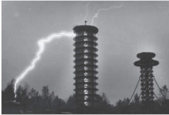
Fig. 3 The photo of the discharges in length of 200 m received on installation VNITZ VEI (Istra) (Photo from site of VNITZ VEI (Istra)).
