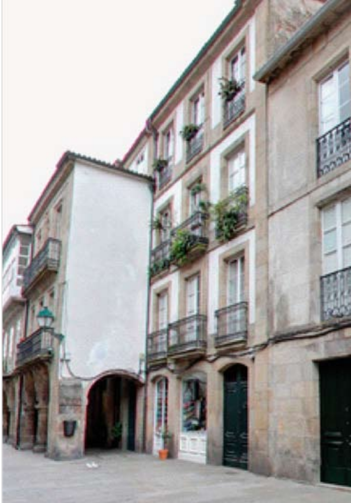
Fig. 5 One of the typical buildings selected as representative
