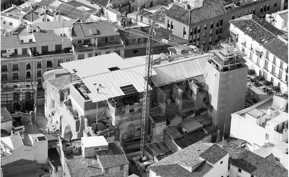
Image 4. Santiago's church, emergency works.(Photograph made by Lorquimur)
