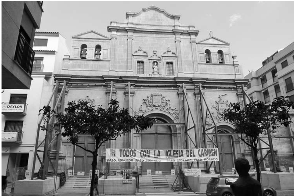
Image 5. Carmen's Church.Stabilization of its main façade
