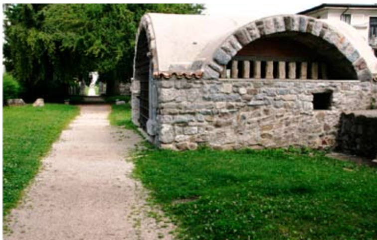
Fig.2. Vaulted lapidary, Indok, MK, foto: G. Zupan
