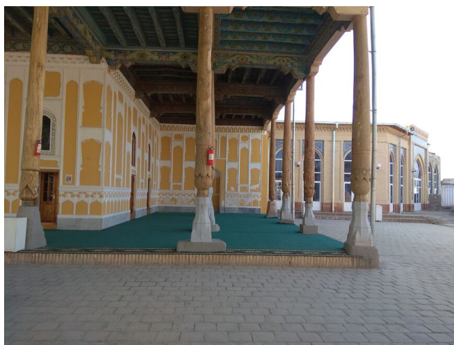
Figure 2. Khoja Zudmurod Mosque (source: http://dkm.gov.uz/uz/mecet-hodza-ziemurod-samarkand )
