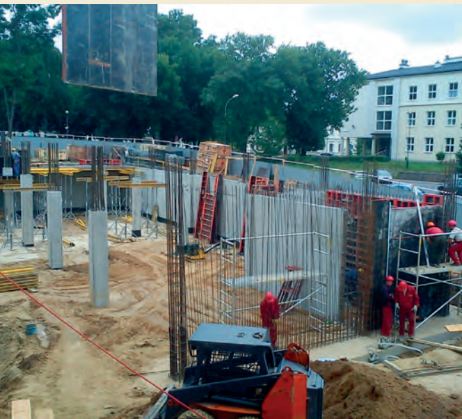
Lipiec 2011 r. – powstaje parking podziemny July 2011 – the underground parking
