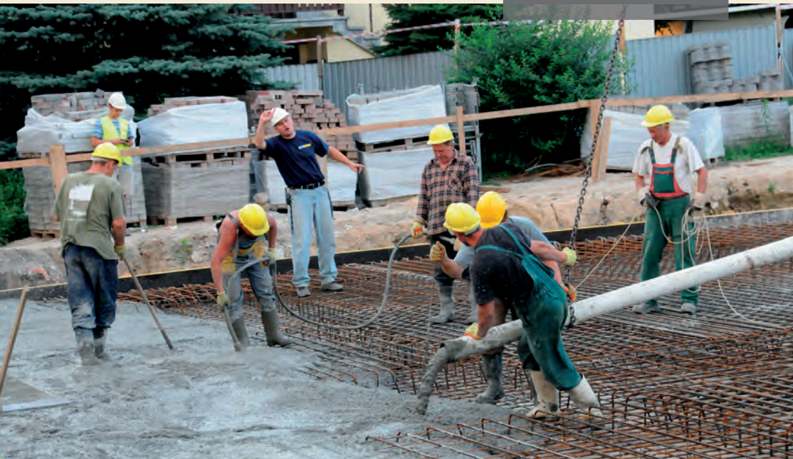
Wylewanie stropu Pouring the concrete floor
