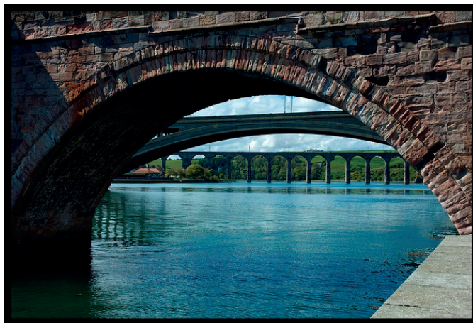
Fot. 6.7.3. Widok amfilady portali bramnych, Royal Border Bridge, Anglia; [I.89]
