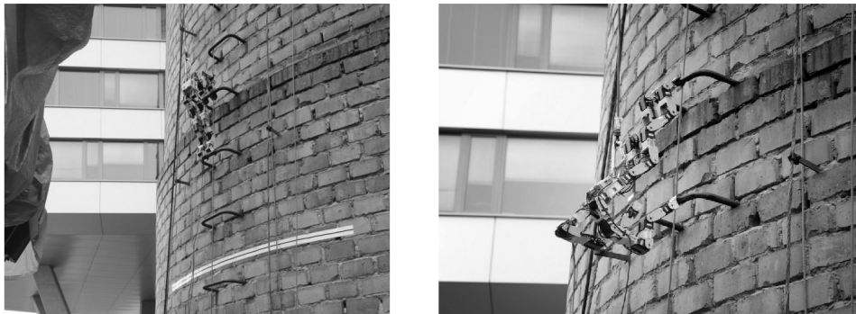
Fig. 5. Test climbing on standpipe chimney ladder [source: own study]
