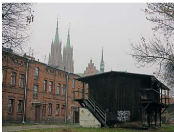
Fig. 74. Economic buildings. Photo by A. Siwek
