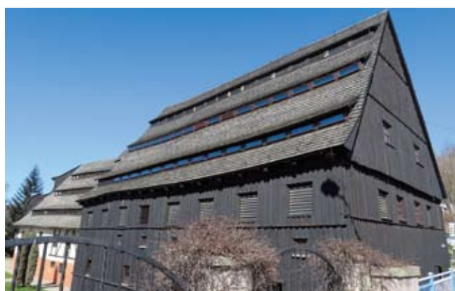
Fig. 11. Drying house facing south-east. Photo by A. Fortuna-Marek
