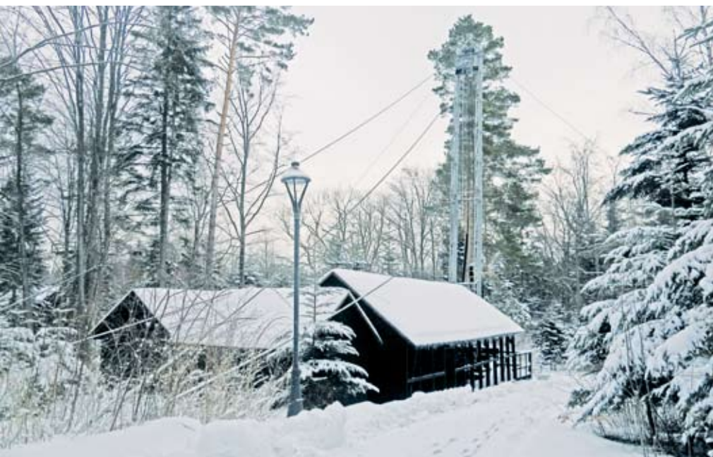
Fot. 34. Relics of the historical cultural landscape of the mine. Photo by A. Siwek
