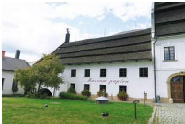
Fig. 60. Paper mill in Velké Losiny. Photo by A. Fortuna-Marek
