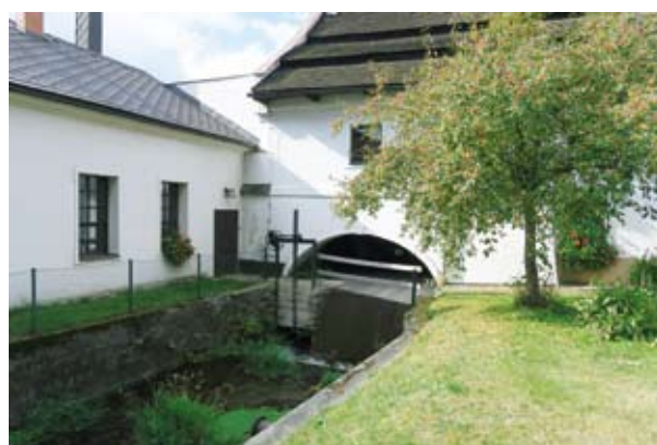
Fig. 63. Paper mill in Velké Losiny. Photo by A. Fortuna-Marek
