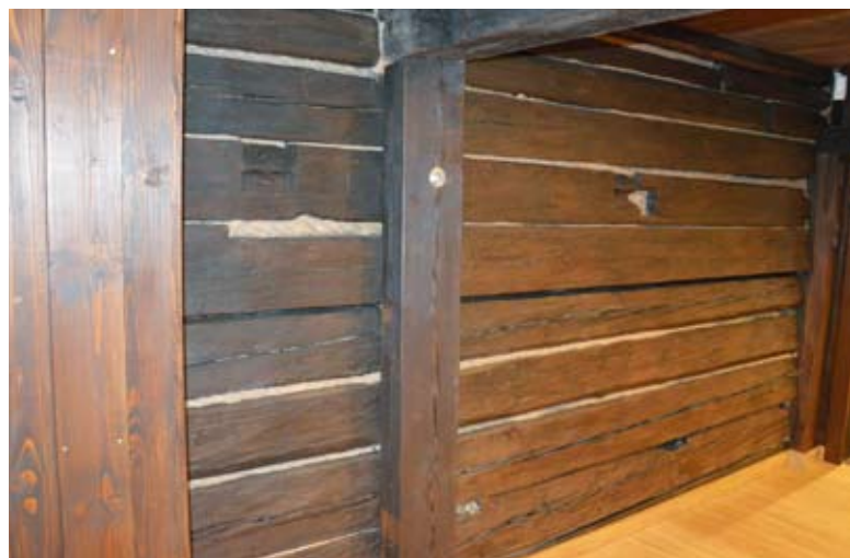
Fig. 52. Log cabin structure of the oldest part of the drying house. Photo by A. Fortuna-Marek
