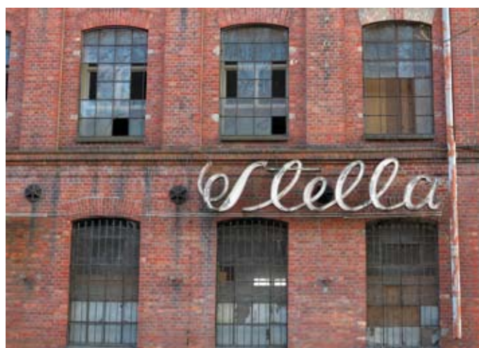
Fig. 61. A fragment of the façade of the building awaiting development. Photo by A. Siwek
