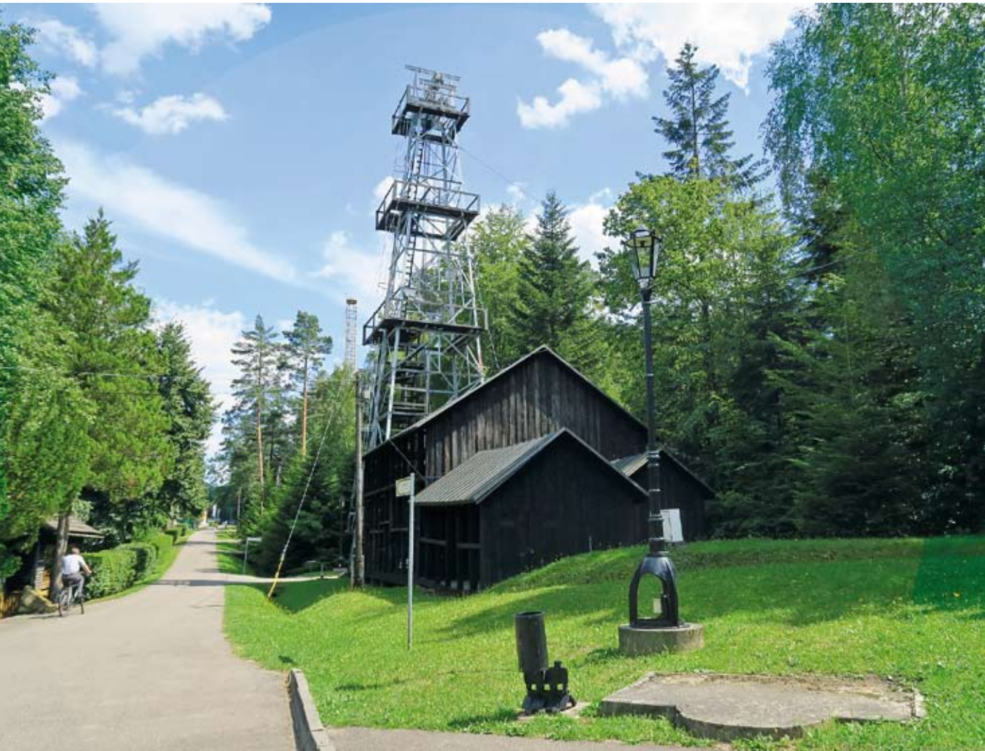
Fig. 56 Drilling rig of the “Bitków” type. Photo by A. Siwek
