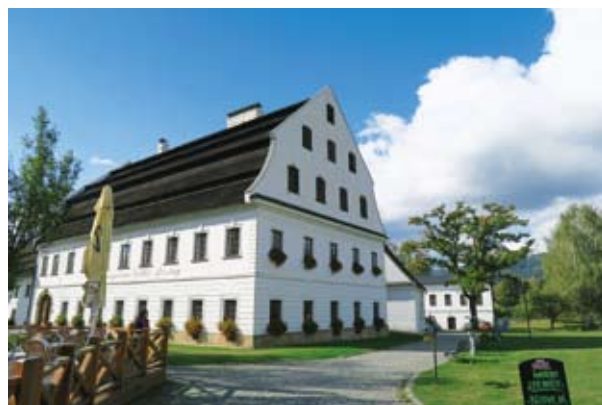
Fig. 61. Paper mill in Velké Losiny. Photo by A. Fortuna-Marek
