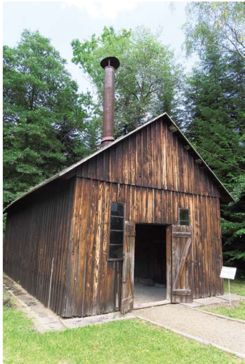
Fig. 43 Boiler room building from 1867. Photo by A. Fortuna-Marek
