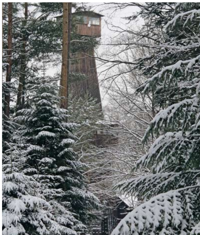
Fig. 54 Polish-Canadian drilling rig. Photo by A. Siwek
