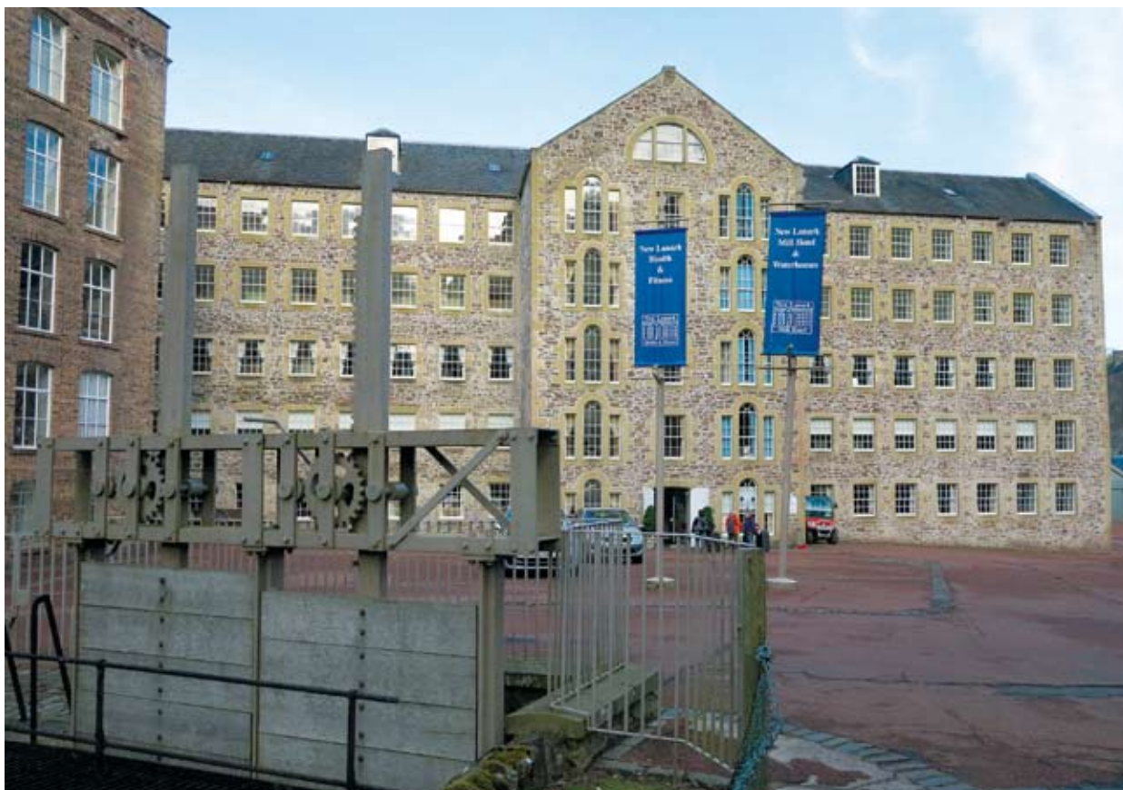
Fot. 79 New Lanark. Factory complex. Photo by A. Siwek
