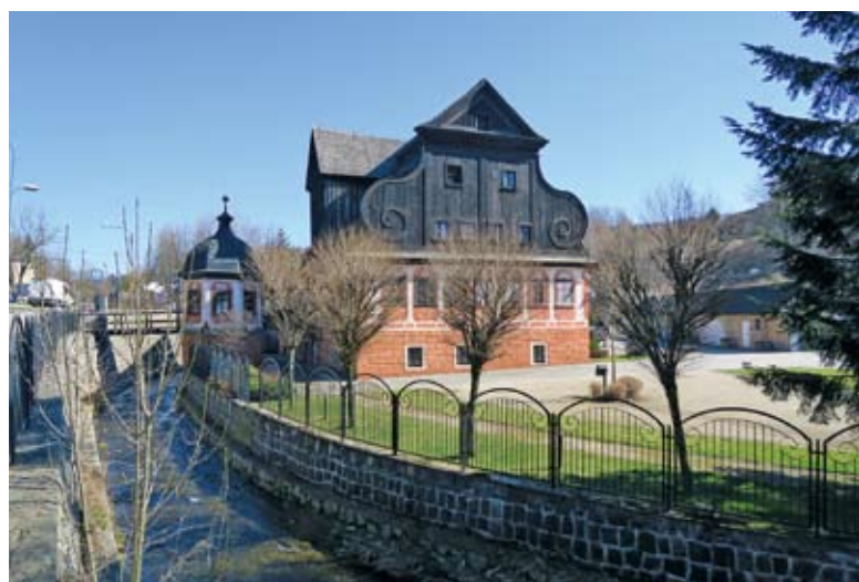
Fig. 9. Paper mill premises. Photo by A. Fortuna-Marek
