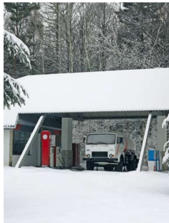
Fig. 61 Fuel station of the "mountain" type, Photo by A. Siwek
