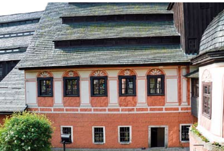
Fig. 22 Part of the north-facing wall. Photo by A. Fortuna-Marek
