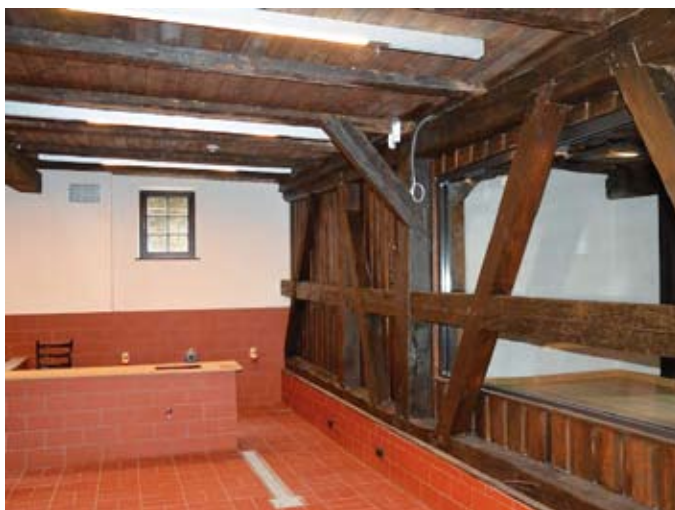
Fig. 42. Drying house – interior after renovation works. Photo by A. Fortuna-Marek
