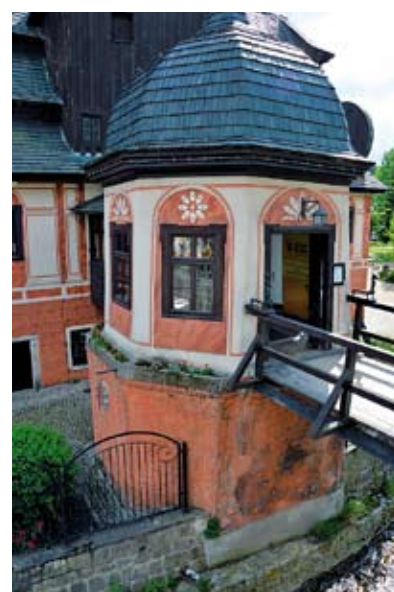
Fig. 34. Entrance pavilion facing north-east. Photo by A. Fortuna-Marek
