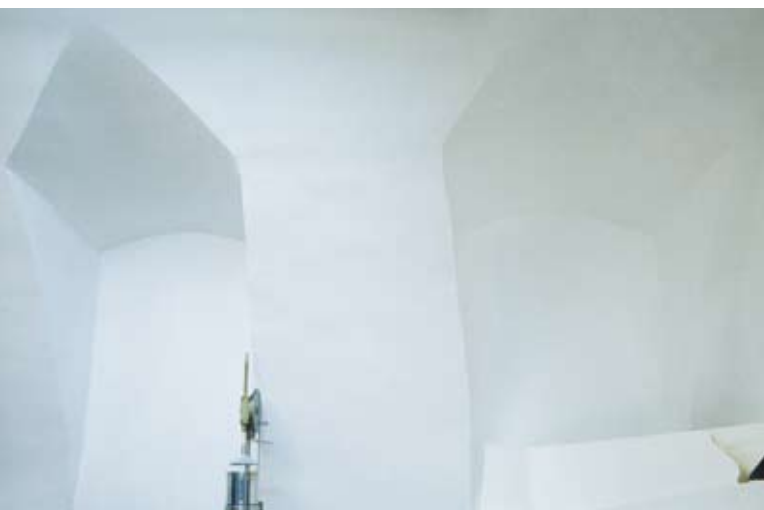
Fig. 49. Paper mill building – barrel vault with lunettes in the lower ground floor. Photo by A. Fortuna-Marek
