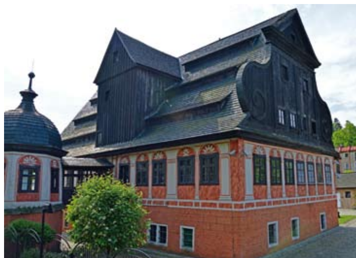
Fig. 21. The paper mill facing north-west. Photo by A. Fortuna-Marek
