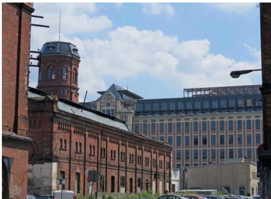
Fig. 72. Industrial architecture. Photo by A. Siwek
