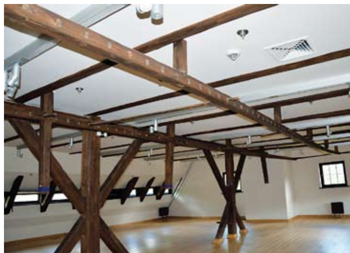
Fig. 43. Drying house – interior after renovation works. Photo by A. Fortuna-Marek
