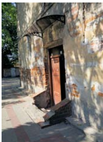
Fig. 57. A fragment of the façade of the building; . Photo by A. Siwek
