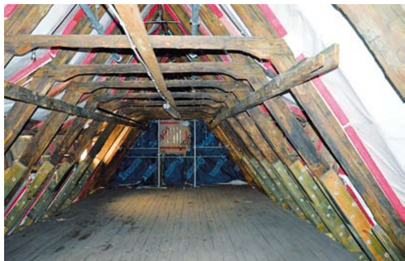
Fig. 50. Roof framework of the paper mill building. Photo by A. Fortuna-Marek
