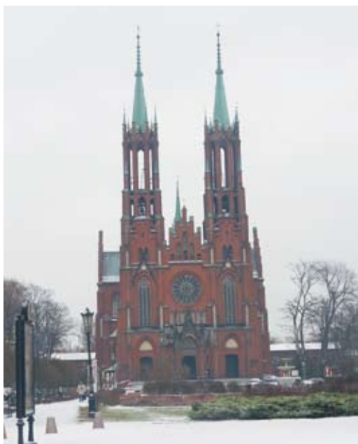
Fig. 71. Monumental architecture – parish church. Photo by A. Siwek
