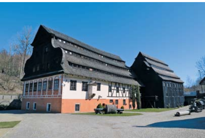
Fig. 8. Paper mill premises. Photo by A. Fortuna-Marek
