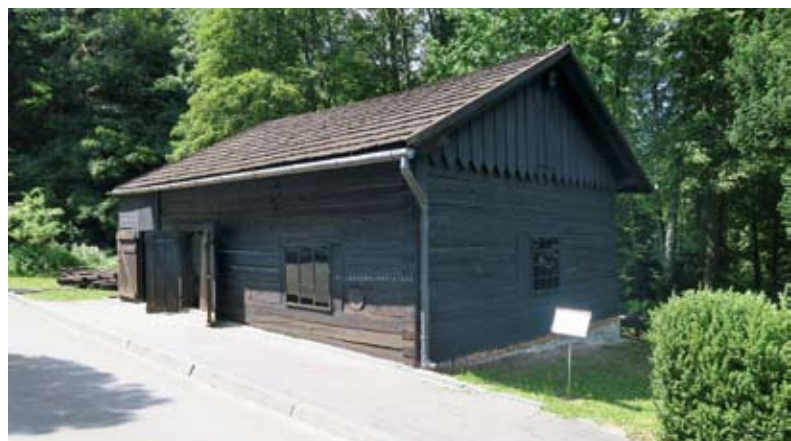
Fig. 36 Workshop building from 1864. Photo by A. Fortuna-Marek
