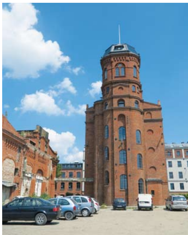
Fig. 46. Factory complex during the revitalization process. Photo by A. Siwek
