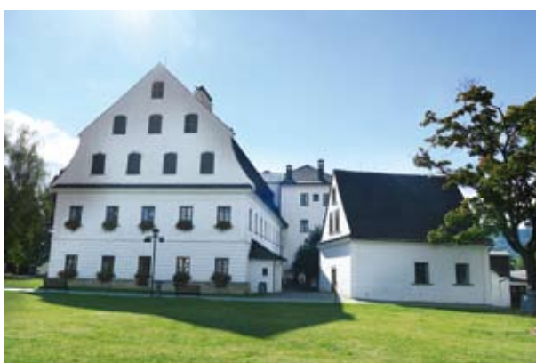
Fig. 62. Paper mill in Velké Losiny. Photo by A. Fortuna-Marek
