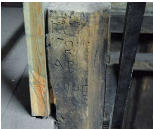
Fig. 51. Staircase structural column in the paper mill building. Photo by A. Fortuna-Marek
