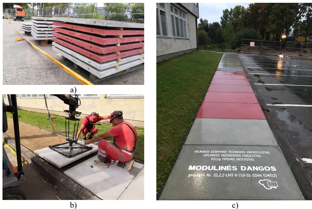
Fig. 1. Prefabricated cement concrete slabs (a), their installation using vacuum lift (b) and constructed pedestrian pathway (c).
