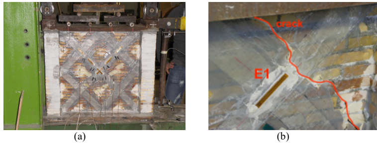
Figure 2. (a) Wall model strengthened with GFRP strips - strain gauges E1,...,E6 on the GFRP strips of main diagonals; (b) view of strengthened side.
